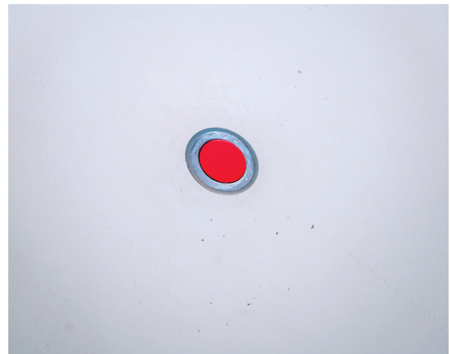
▶ Steel-clad tying aperture with sealing cone
